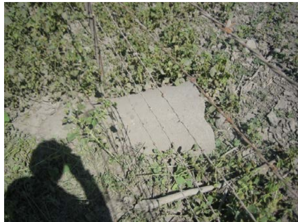
Photo C-4 Culvert Inlet for the Overflow Channel (Historical Mariposa Slough channel)
