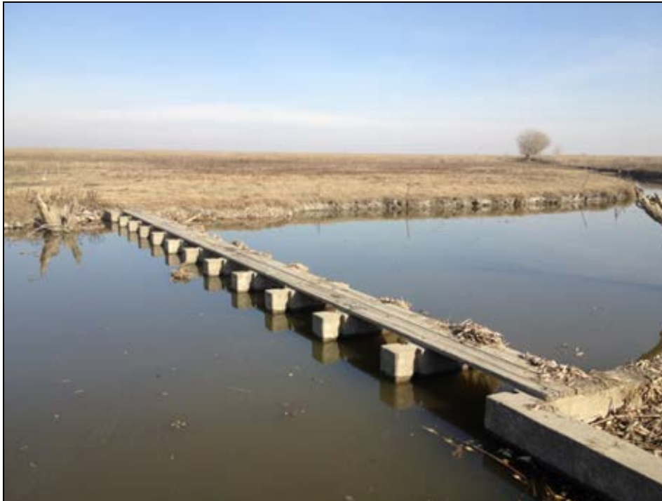
Photo 4 Upper Merced Weir Looking Downstream toward the East (Right) Bank
