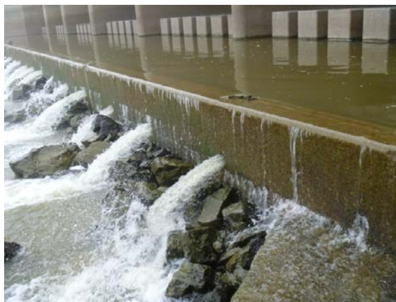
Photo B-4 Downstream Sill and Rip Rap Located at the Structure Outlet
