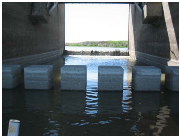
Photo B-2 Structure Bay with Baffles Looking Upstream from Bay Outlet
