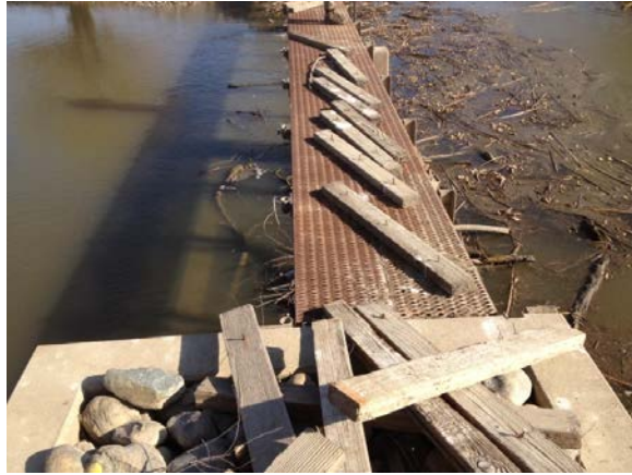
Photo D-2 Lower Merced Weir Metal Grate with Wooden Boards
