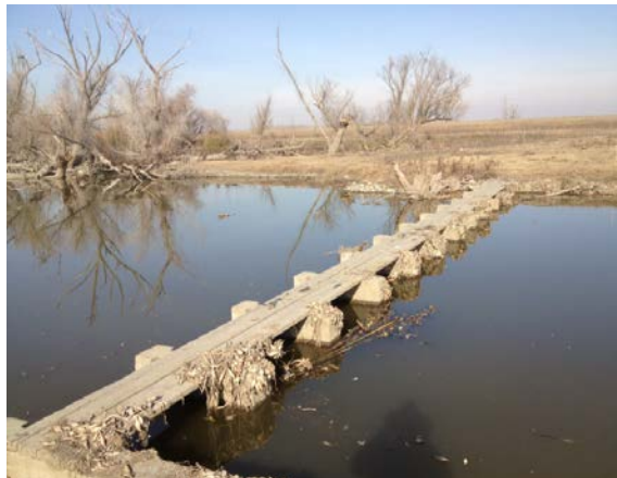
Photo D-6 Upper Merced Weir Looking Downstream
