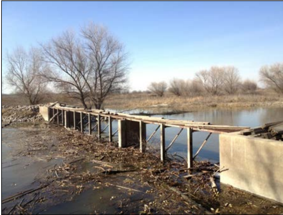
Photo 3 Lower Merced Weir Looking Downstream Toward the West (Left) Bank
