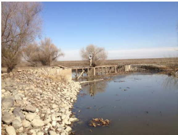
Photo D-3 Lower Merced Weir Upstream Looking Downstream from Cobble Bank
