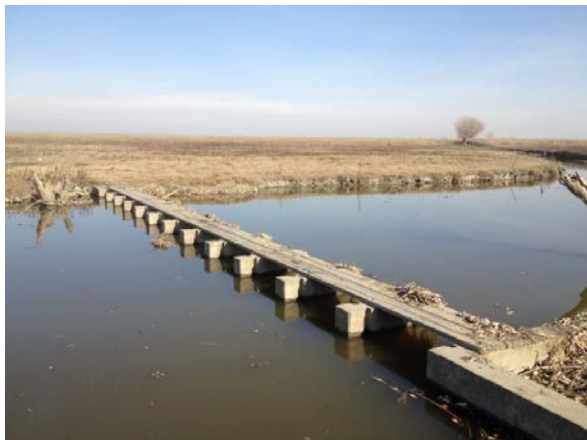
Photo D-5 Upper Merced Weir Looking East at the Right Bank
