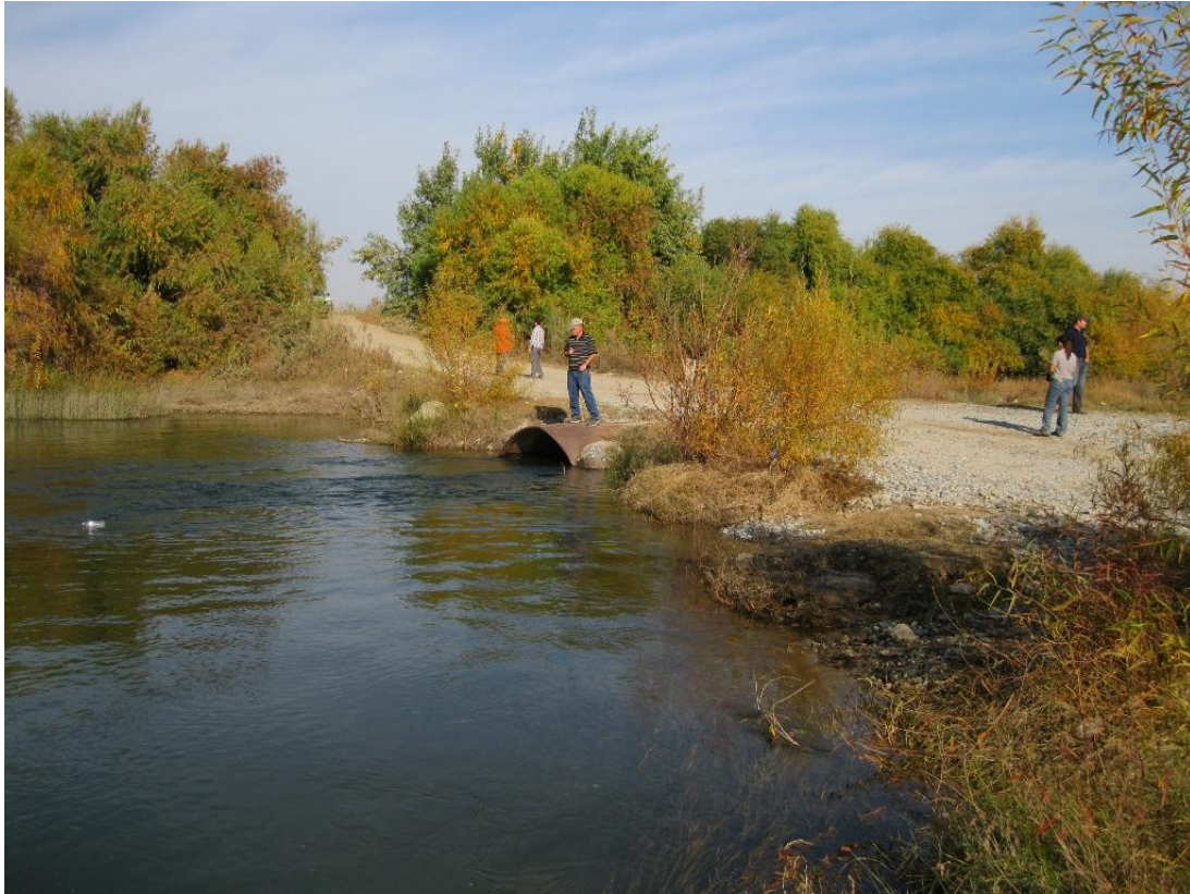
Figure 17. San Mateo Crossing from the left bank
