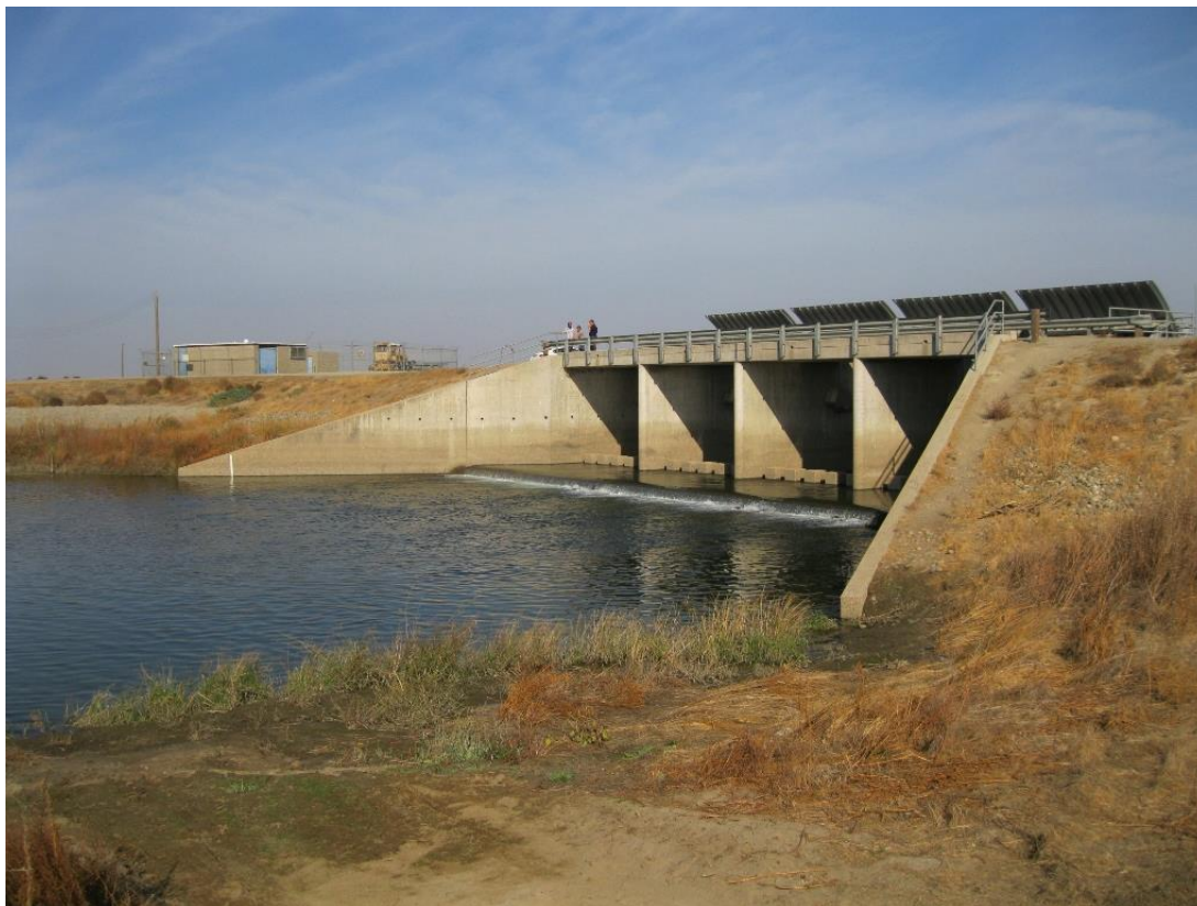
Figure 16. On-river portion of the Chowchilla Bifurcation Structure from the left bank
