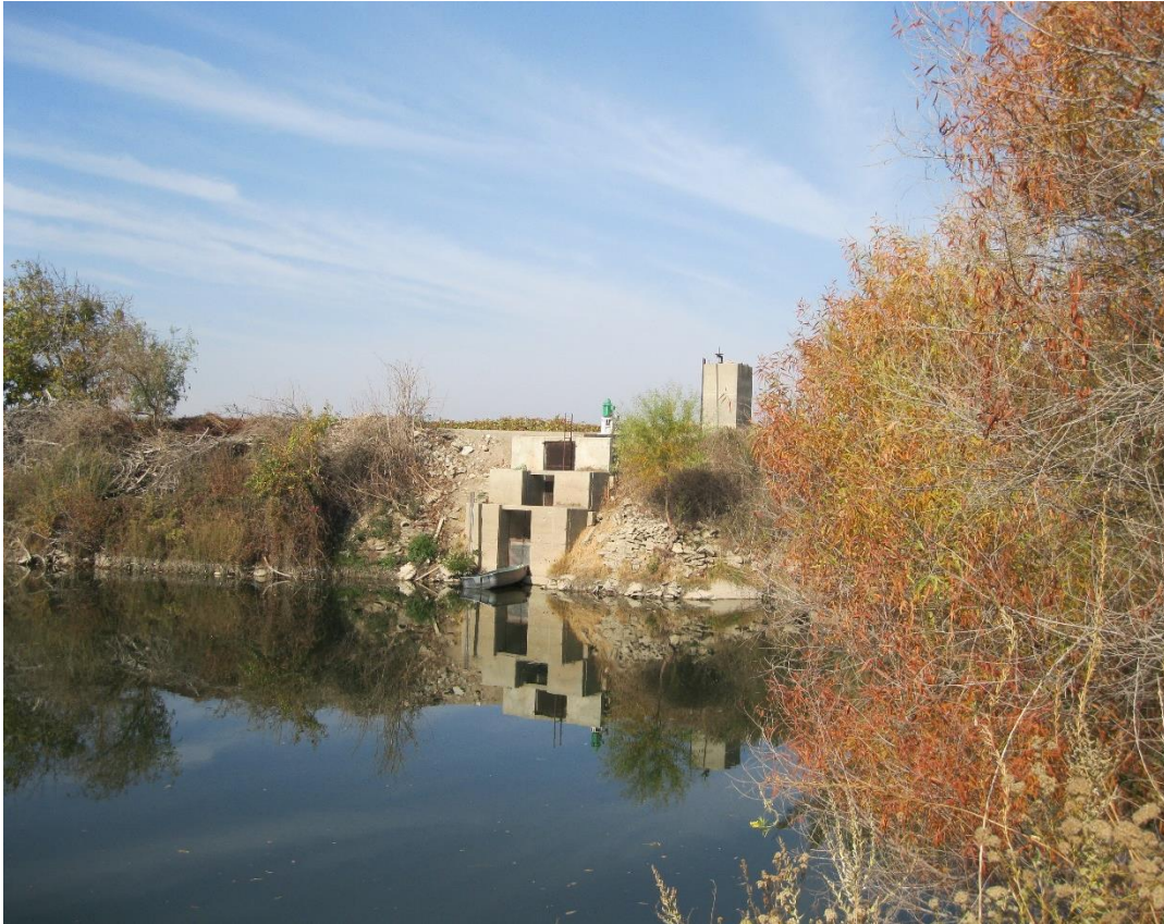
Figure 15. Emmert Pump Station from the left bank
