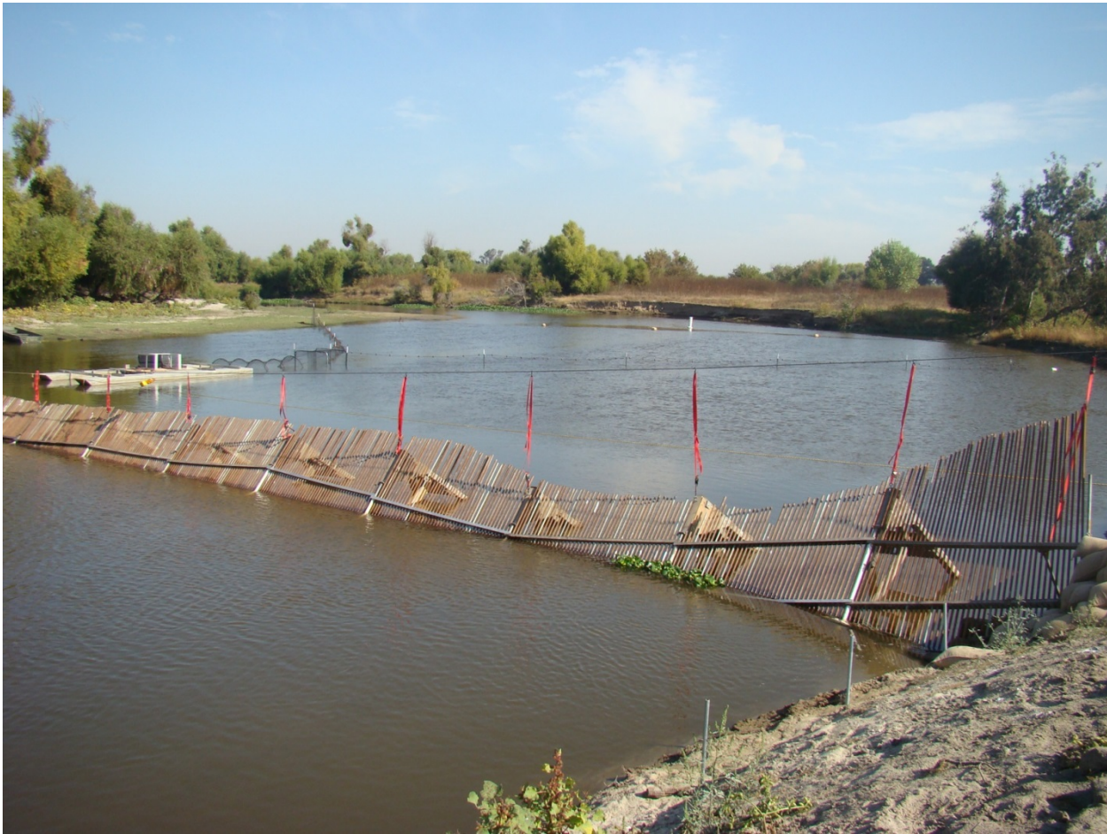
Figure 6: fyke trap with floating trap downstream of Hills Ferry Barrier
