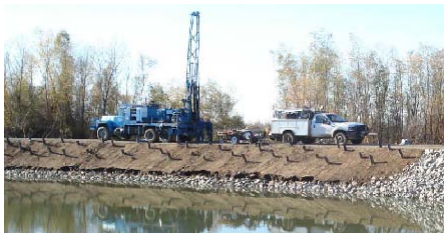
Drill Rig and support vehicle for HSA/SPT Borings
