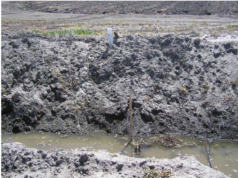
Photo #4: Open drain with stagnant water and staff gage (4/7/10).
