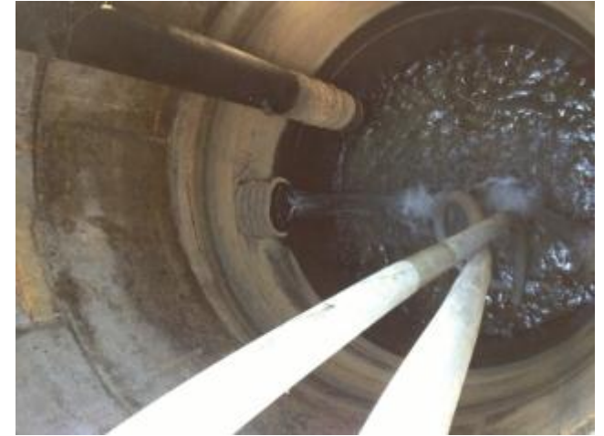
Drain Sump, Submersible Pump
