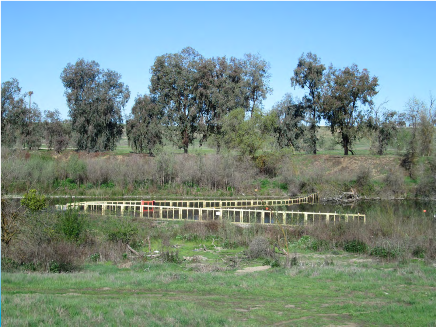
Fish Collection Weir near Highway 41 DRAFT – For Discussion Purposes Only
