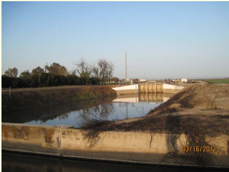
Arroyo Canal Headworks
