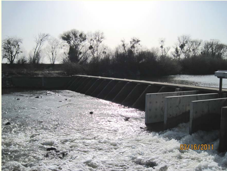
Sack Dam (March 2011)
