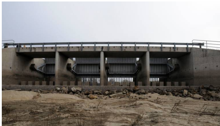
Figure 1-6 View from downstream of the Chowchilla Bifurcation Structure in Reach 2B
