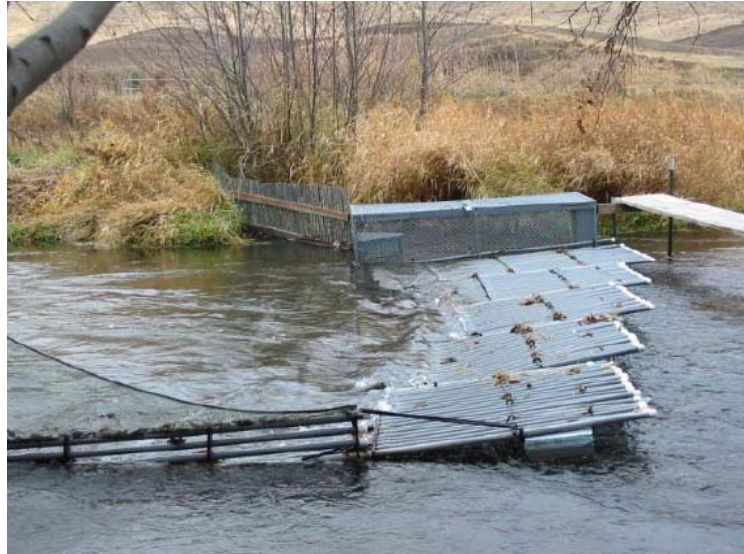
Figure 7-7 Application of a Floating Picket Weir
