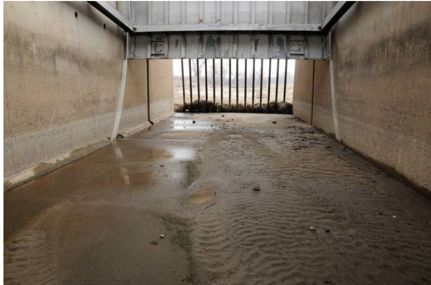
Figure 1-7 Inside of one of the bays at the Chowchilla Bifurcation Structure 1
