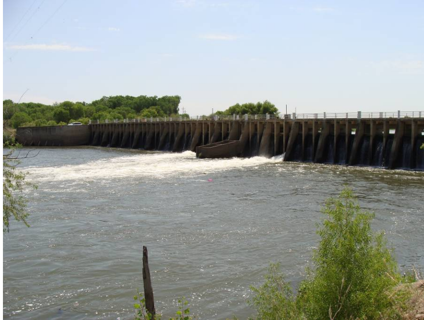
Figure 1-11 Downstream face of Mendota Dam
