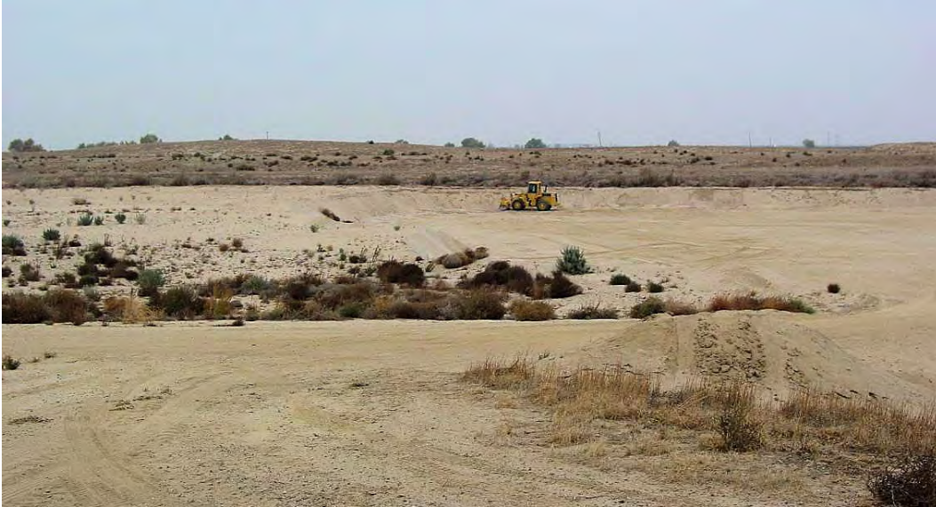
Figure 14-14. View of 200,000 Cubic Yard Sediment Trap in the Chowchilla Bypass just Downstream from the Chowchilla Bifurcation Structure
