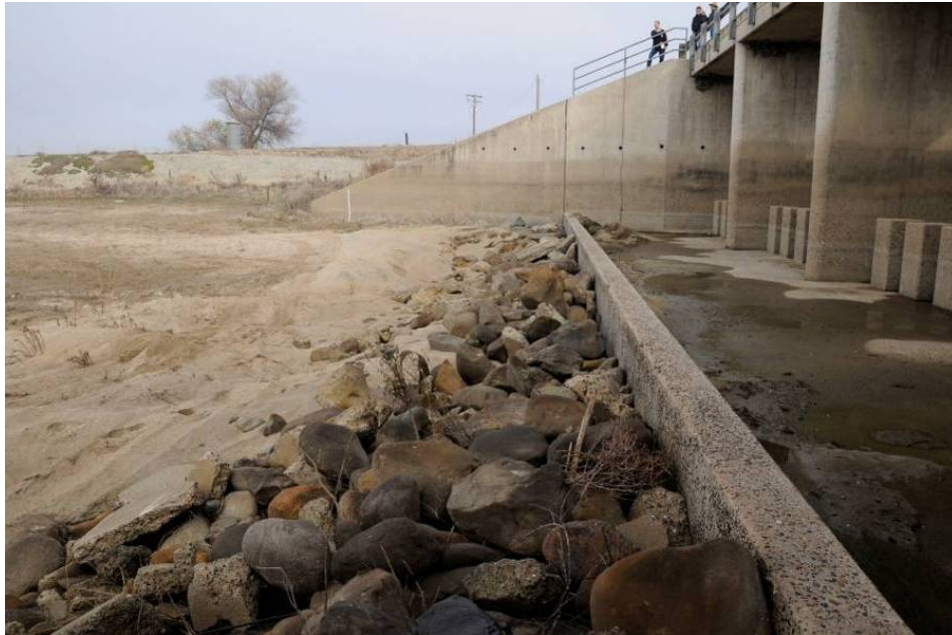
Figure 1-6. Concrete sill and bordering riprap along the downstream edge of the Chowchilla Bifurcation Structure in Reach 2B 2 (12/15/09)
