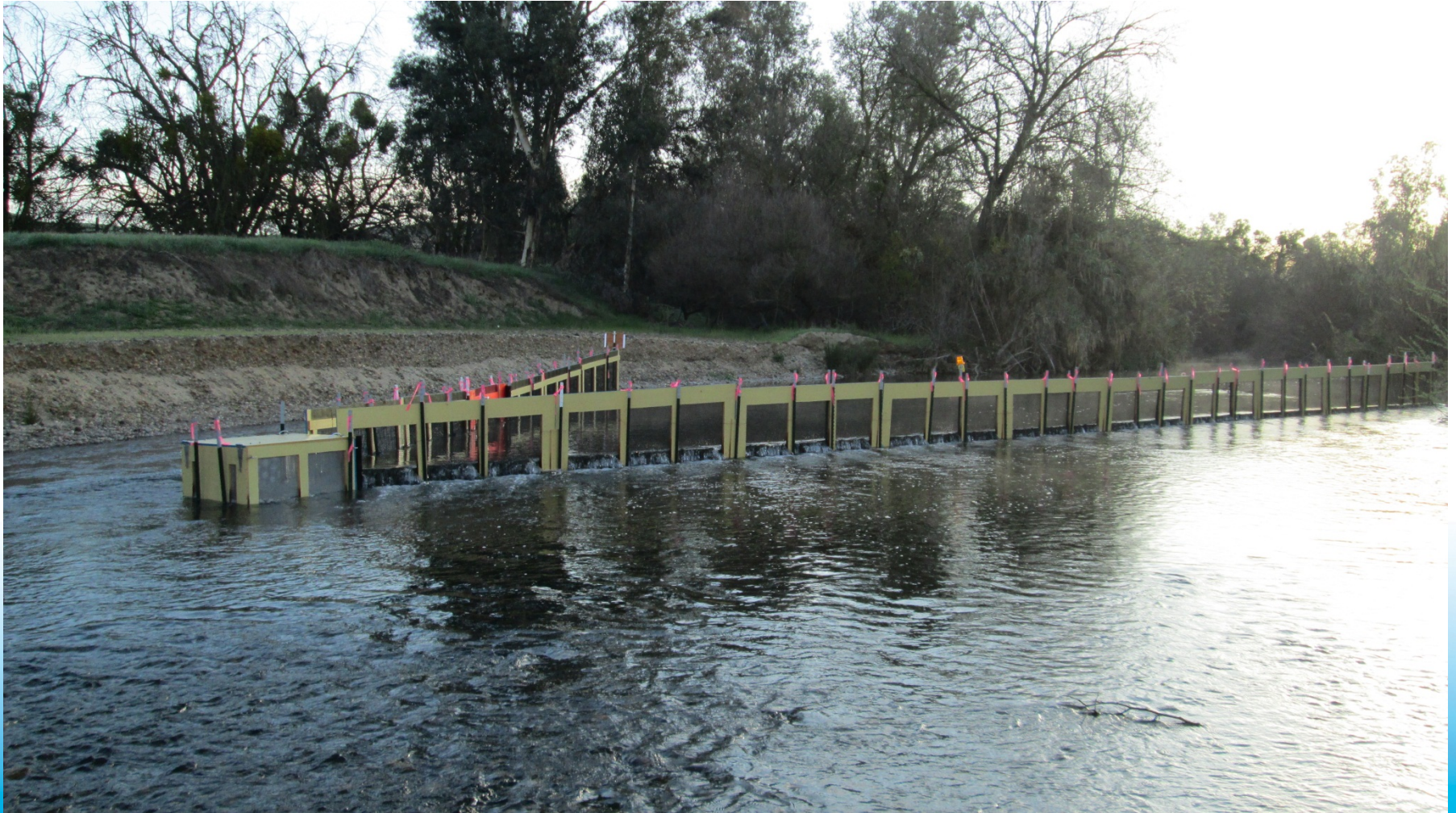
Fish Collection Weir at Scout Island
