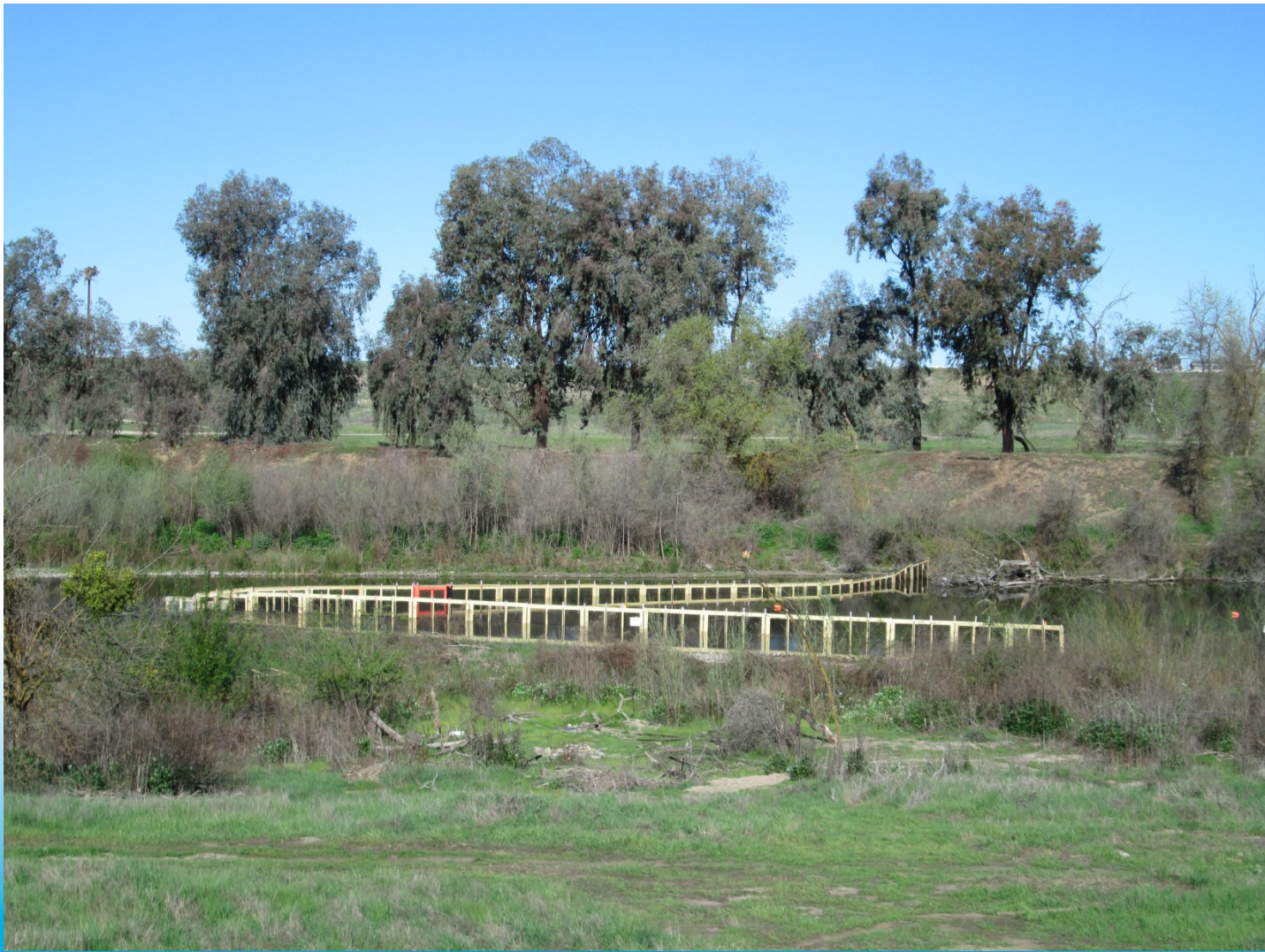
Fish Collection Weir near Highway 41
