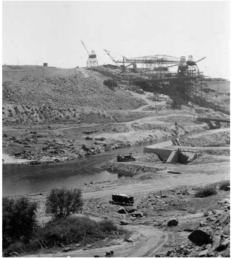
Friant Dam Construction
