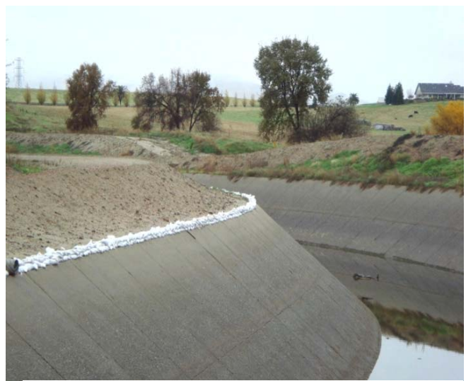
Sandbags placed on FKC to restore capacity
