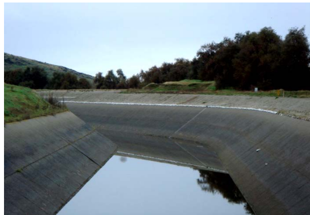
Sandbags placed on the FKC to restore capacity
