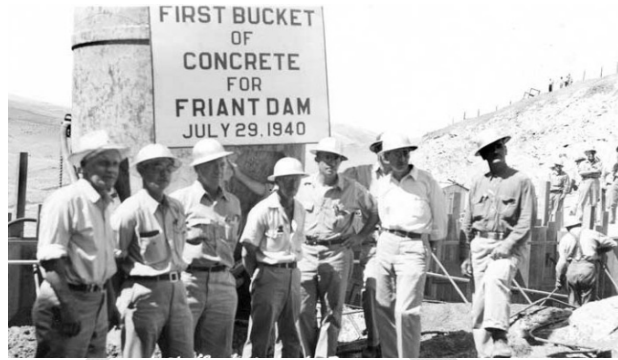
Friant Dam construction
