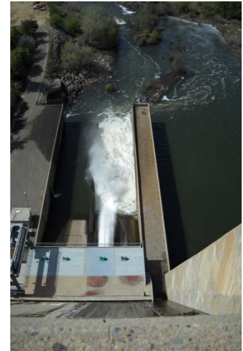
Friant Dam river outlets
