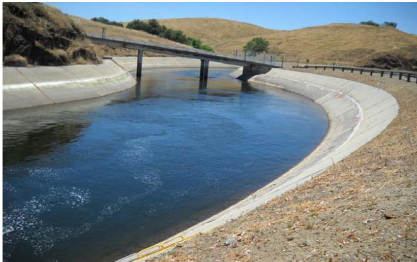
FKC downstream of Friant Dam
