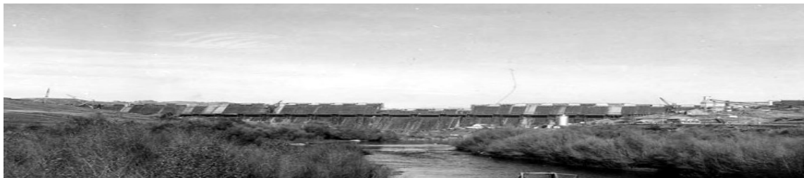
Friant Dam Construction
