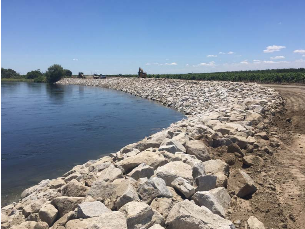
Figure 11-3. Photo of Erosion Site After Repairs Were Completed (looking upstream)
