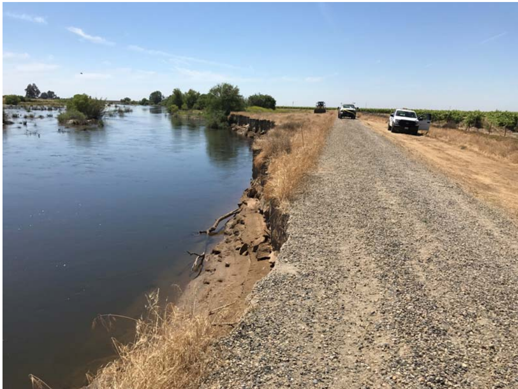
Figure 11-2. Photo of Erosion Site Prior to Repairs (looking upstream)
