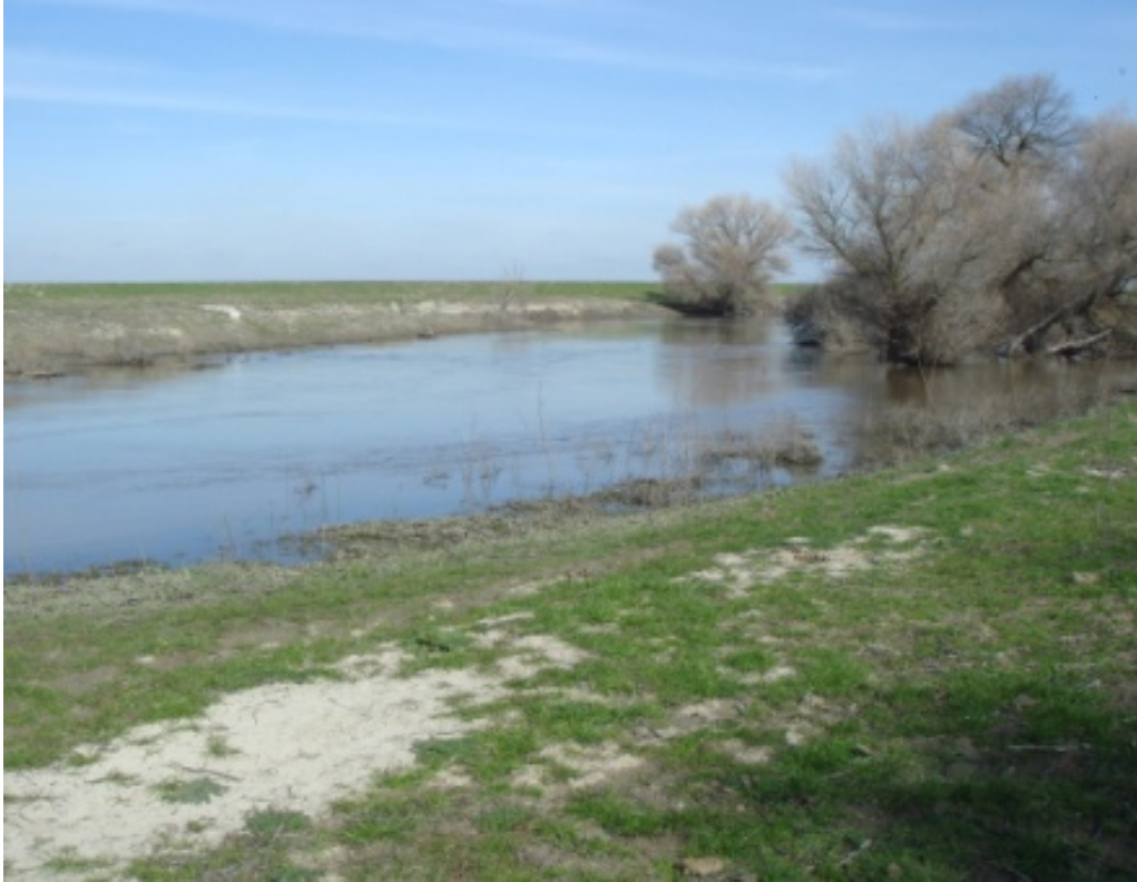
Figure 9-12. Lower Eastside Bypass, upstream of Bear Creek Confluence.
