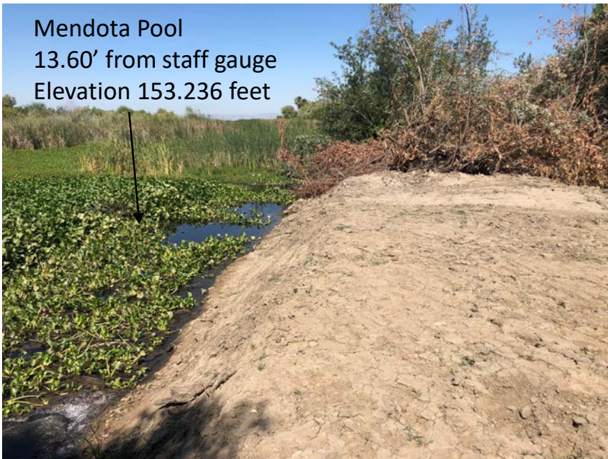
Photographs of the recent plug constructed to repair the outer berm and stop Seep #2.
