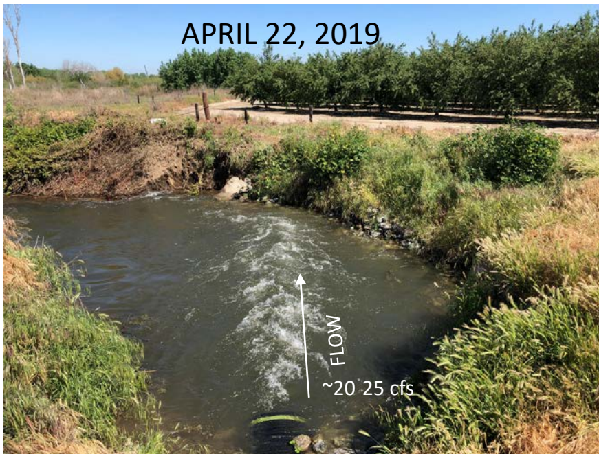
Photo 2 Looking north at the discharge area of the drainage ditch. The HDPE pipe crosses beneath Columbia Road in the northwest corner of the property and was recently modified with a 45° bend to direct any future flow away from the armor lined embankment.
