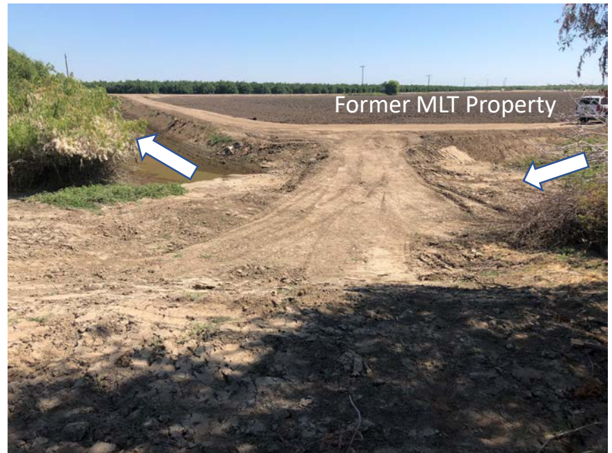
Photographs of the recent plug constructed to repair the outer berm and stop Seep #2.
