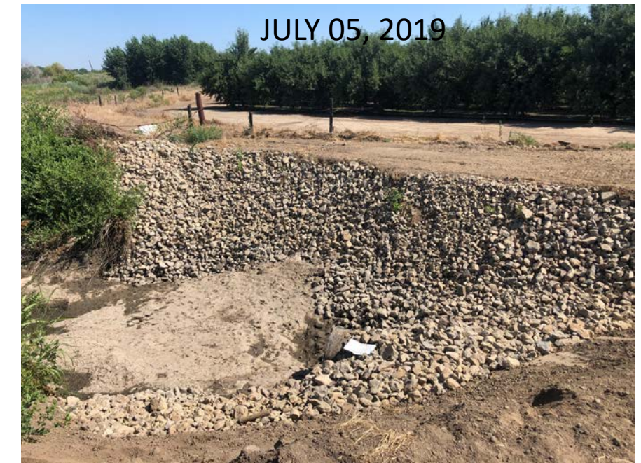
Photo 2 Looking north at the discharge area of the drainage ditch. The HDPE pipe crosses beneath Columbia Road in the northwest corner of the property and was recently modified with a 45° bend to direct any future flow away from the armor lined embankment.
