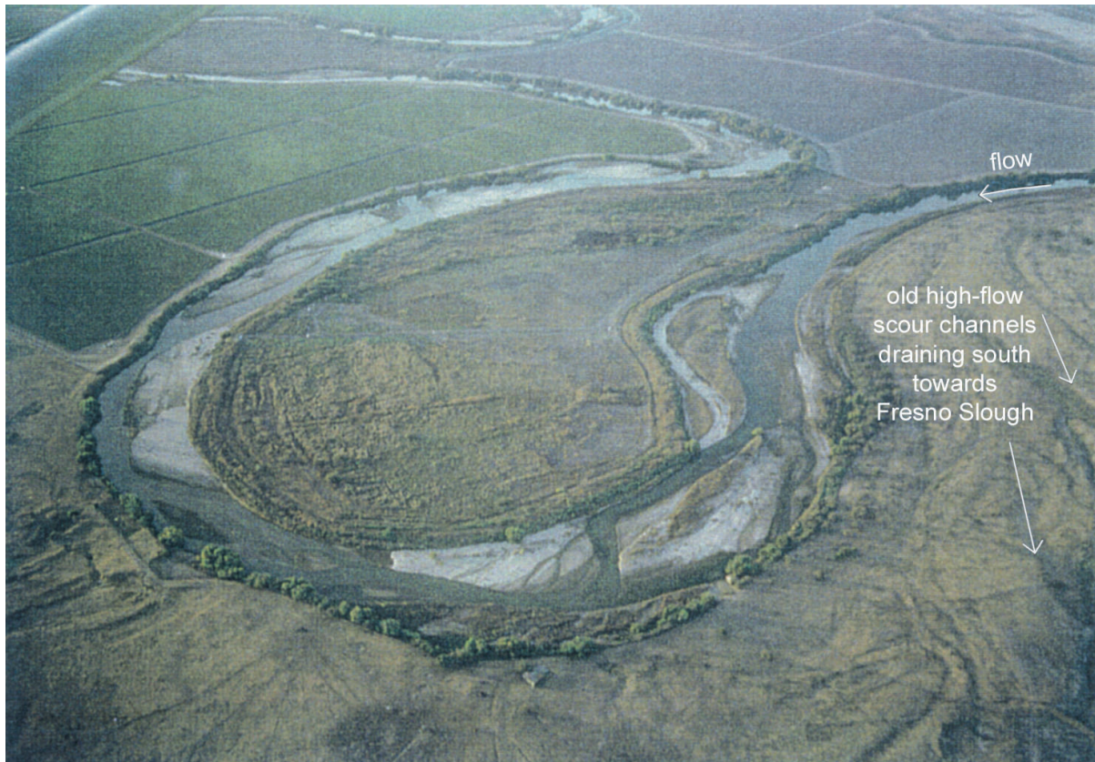
Figure 3-34. View looking downstream of a high amplitude bend in the San Joaquin River in Reach 2B (RM 215). Channel capacity is reduced by sediment deposition in the bed of the channel. Within-levée design capacity within this reach of the river is about 2,000 cfs. This reach is usually dry most of the year. From JSA and MEI (1998).
