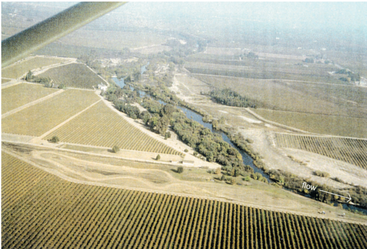
Figure 3-28. View upstream of the San Joaquin River at about RM 237. The channel is bounded by alluvial terraces, and has not been mined for sand and gravel in this specific location. From JSA and MEI (1998).
