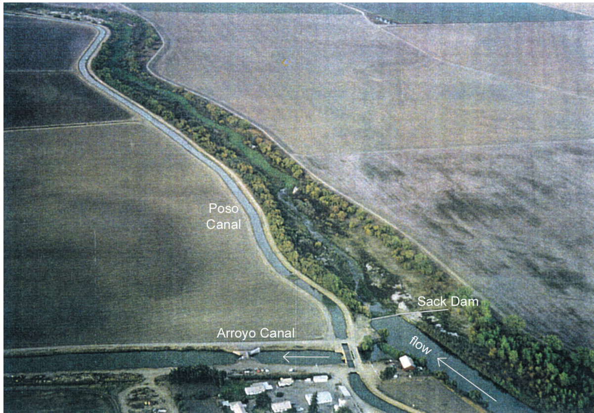
Figure 3-41. View looking downstream of Sack Dam and the headgates for the Arroyo Canal at RM 182. The dam is the terminus for Delta-Mendota water conveyed down the San Joaquin River. The Poso Canal parallels the river on the left bank. From JSA and MEI (1998).
