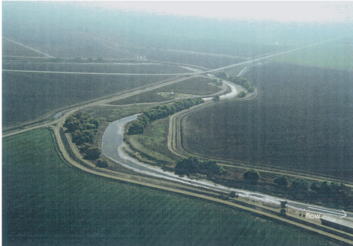
Figure 3-51. View looking upstream at the San Joaquin River at Turner Island Road crossing, RM 157. Design capacity of the channel and levees is about 1,500 cfs; however, actual capacity in many portions of this reach is much less. From JSA and MEI (1998).
