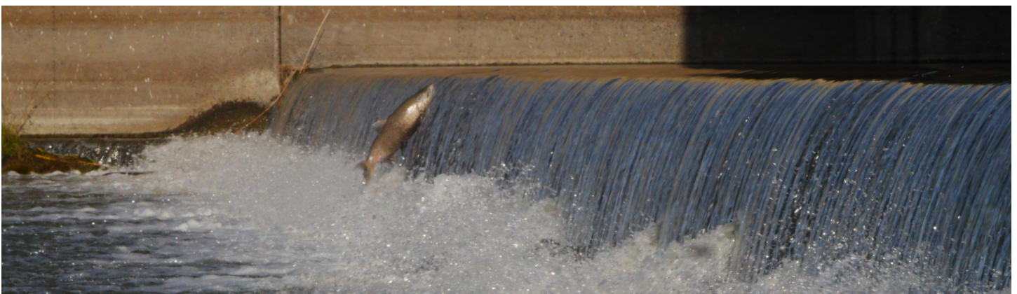
Salmon jumping at the Eastside Bypass Bifurcation Structure.
