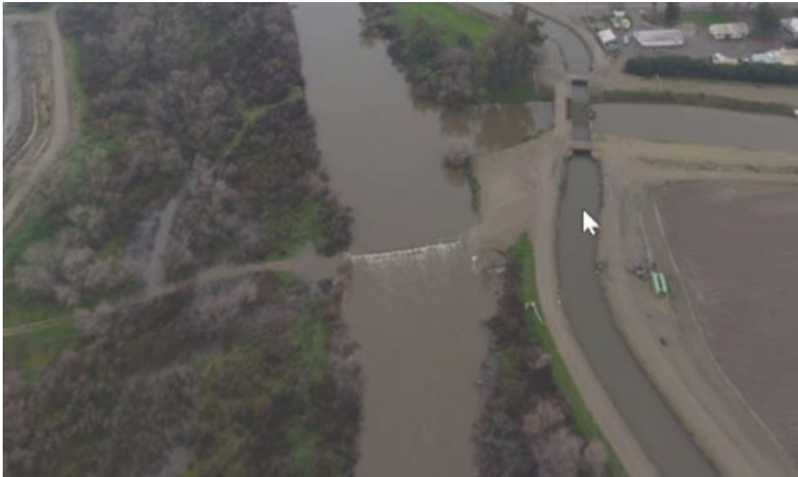
Figure 1 - Flood flow, approximately 3500 cfs. Flashboards and gates have been removed. Notice flood flow outflanking the structure to the left of the dam.
