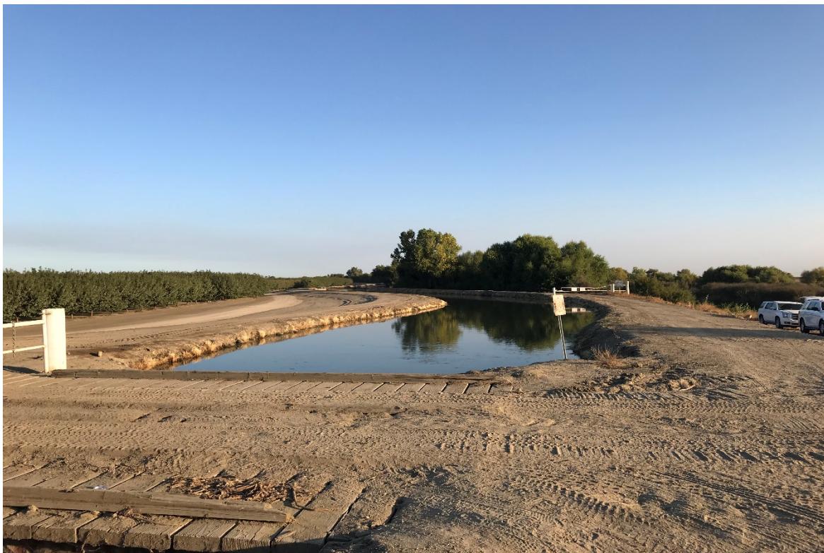
Figure 3 – Poso Canal looking north, adjacent to San Joaquin River and Sack Dam
