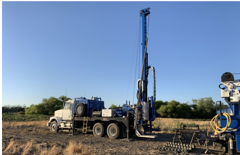
Reclamation drill rig
