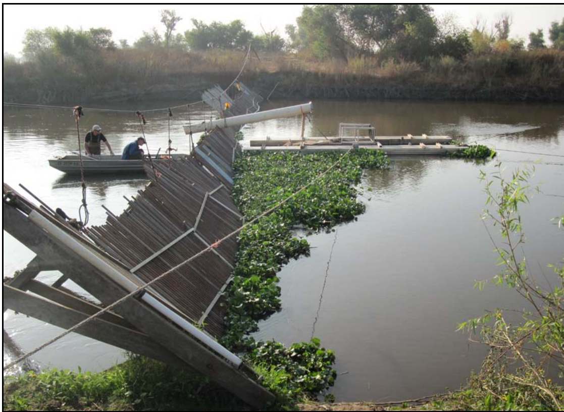
Figure 1.—Hills Ferry Fish Barrier and fish trap on the San Joaquin River, California.
