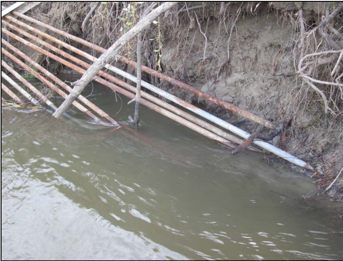
Figure 12.—Gaps in the conduit pickets can provide passage for adult Chinook salmon beyond the Hills Ferry Barrier.
