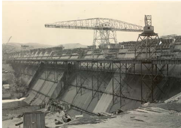
Friant Dam Under Construction
