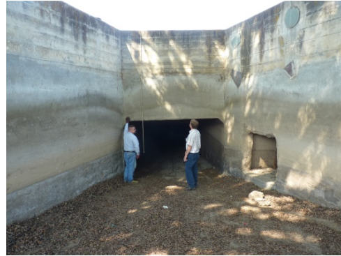
Tulare ID's Kaweah River Siphon
