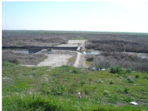
Sand Slough Control Structure. Photo: USFWS, San Joaquin Restoration Program
