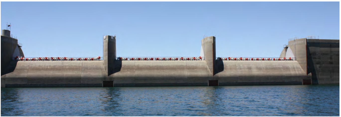
Friant Dam view from Millerton Lake side
