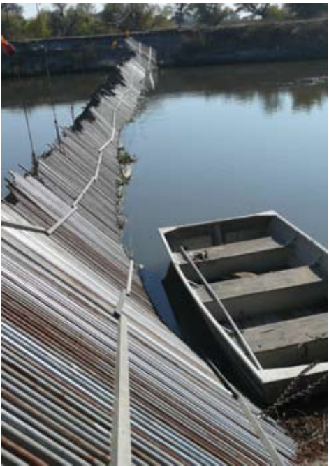
The Hills Ferry Barrier is installed every fall to prevent Merced River salmon from straying up into the San Joaquin River
