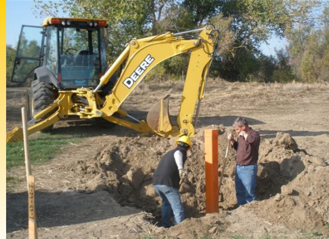
Installation of a monitoring well
