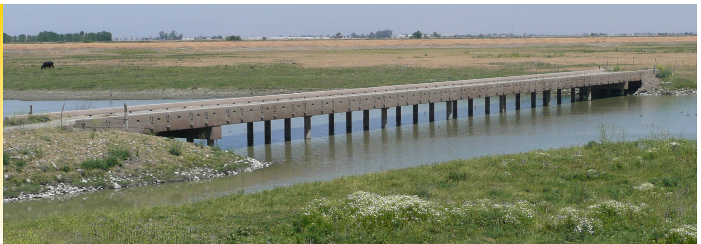
Eastside Bypass Bridge
