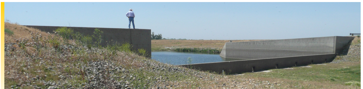
Mariposa Bypass Drop Structure
