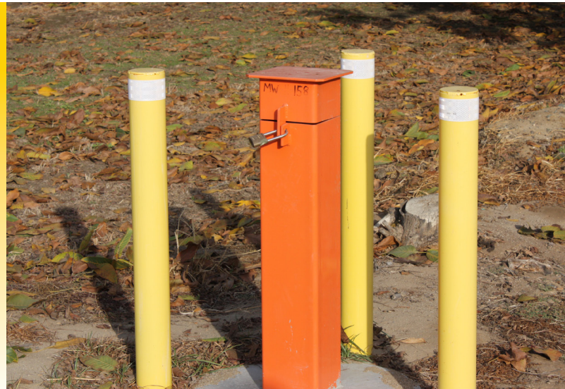
A newly installed monitoring well
