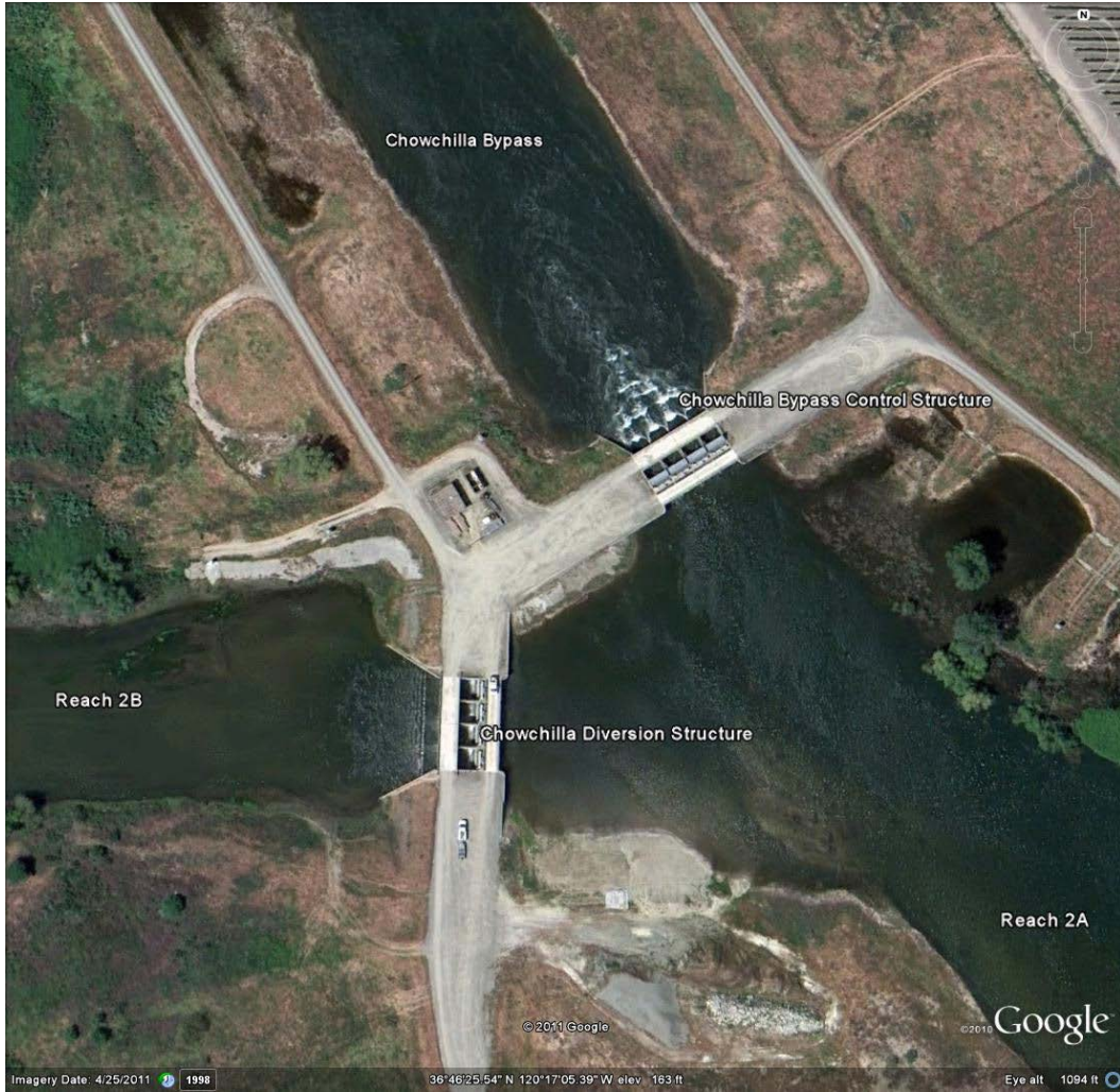
Figure 3-7. Aerial view of the Chowchilla Bifurcation Structure (CBS).
