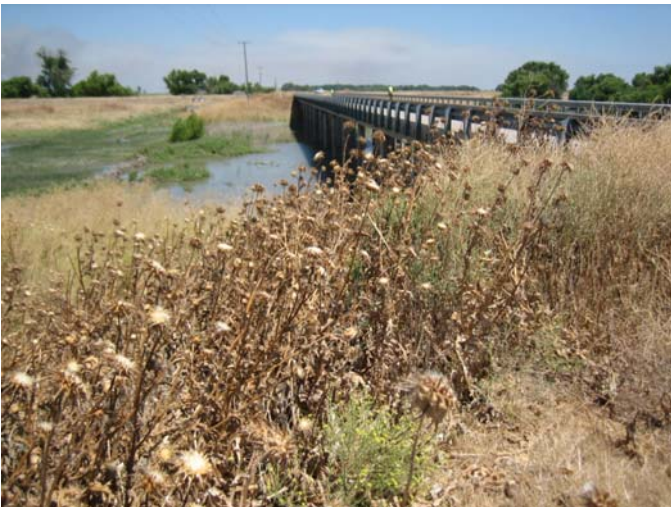
Photo 52_A. Sandy Mush Road Bridge looking downstream
