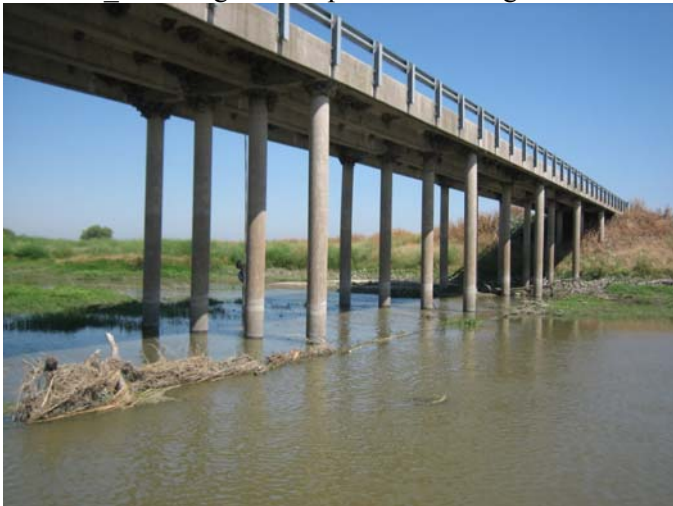
Photo 44 A. Bridge from upstream looking downstream
