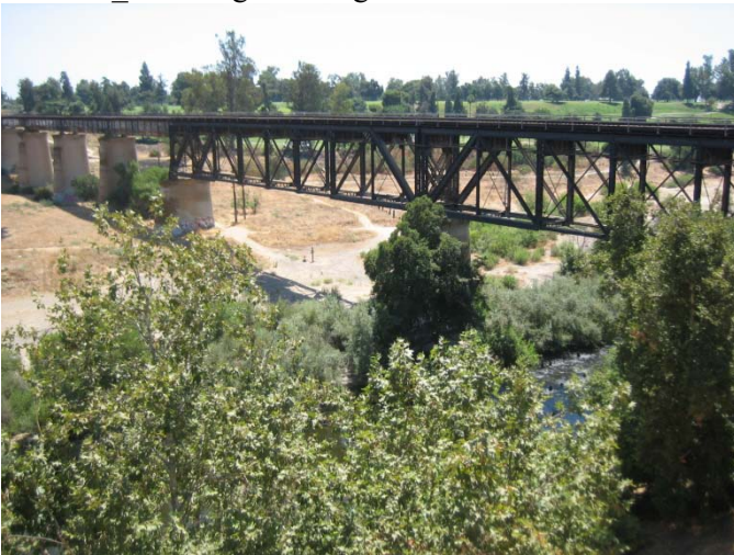
Photo 14_A. Bridge looking downstream
