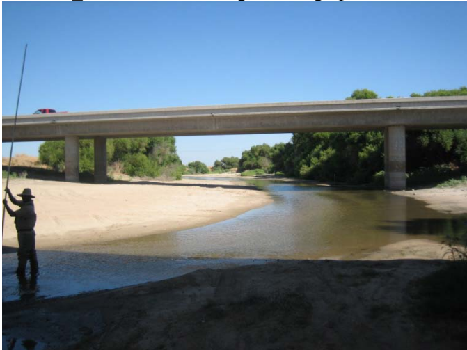
Photo 27_A. Eastbound bridge looking upstream
