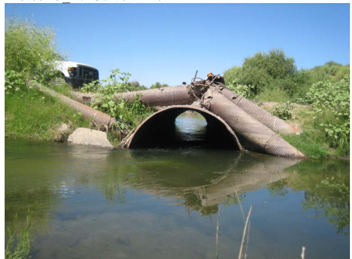
Photos 23_B. Culvert inlet
