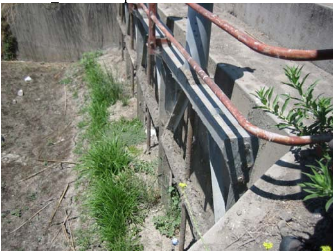
Photo 28 A. Gates upstream
