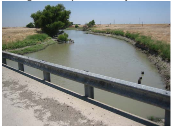
Photo 47_B. Channel upstream from bridge deck
