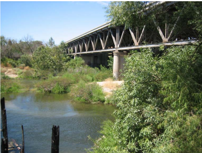
Photo 16_A. Bridge looking upstream
