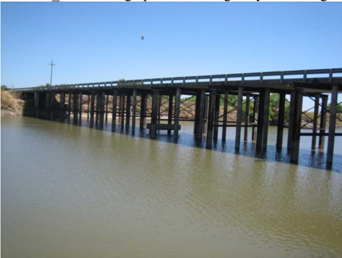
Photo 42_A. Looking upstream at Highway 165 Bridge
