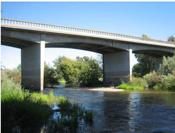
Photo 10_A. Bridge looking upstream
