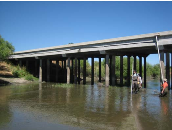
Photo 43_A. Looking downstream at Highway 140 Bridge, left bank
