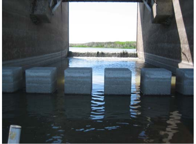
Photo 48_B. Downstream looking upstream from end of bay
