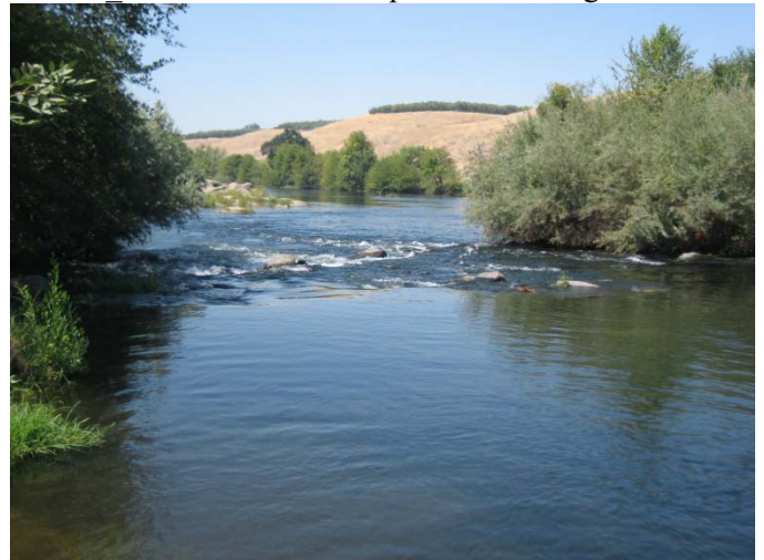
Photo 4_B. Rock weir from upstream looking downstream
