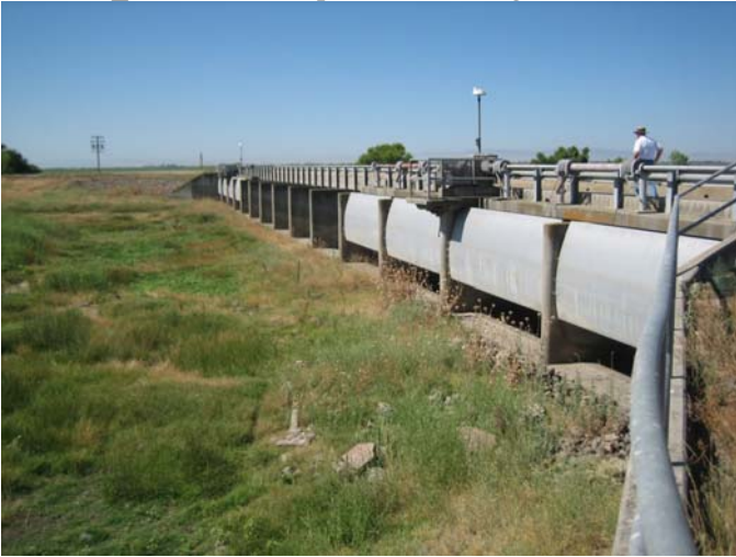
Photo 49_A. Structure,upstream looking downstream
