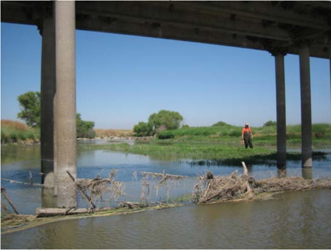
Photo 44 A. Channel looking downstream
