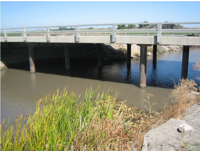
Photo 32_A. Bridge, upstream looking downstream
