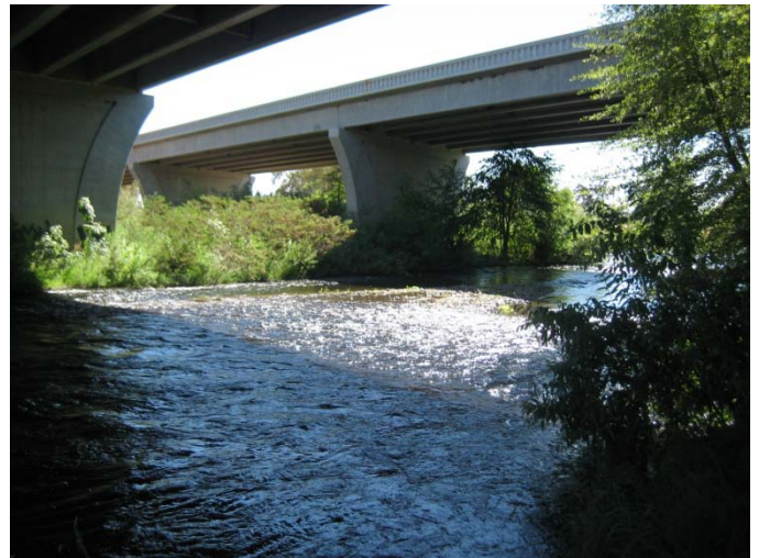
Photo 11_B. Channel between bridges looking downstream
