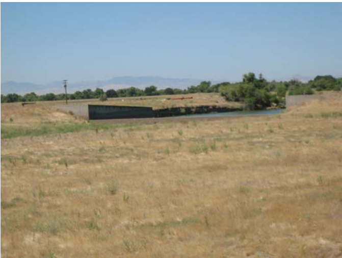
Photo 35_A. Structure, upstream looking downstream
