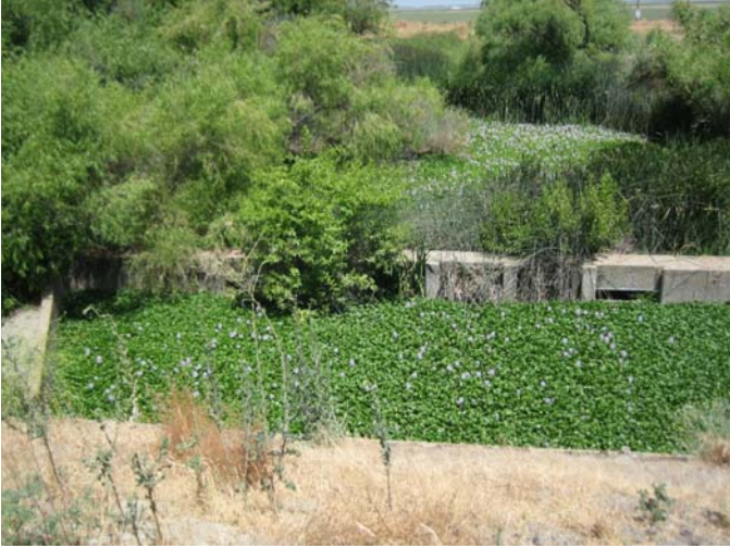
Photo 28_C. Weir downstream culvert outlets, channel looking downstream
