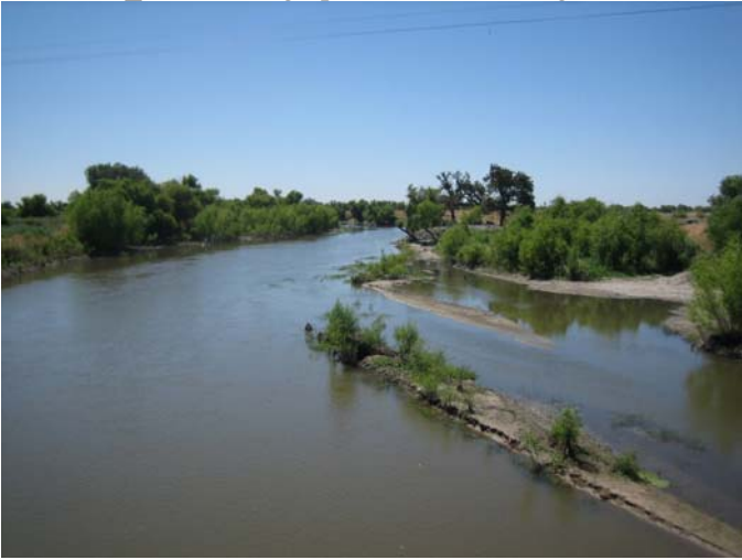
Photos 43_C. Looking upstream from bridge
