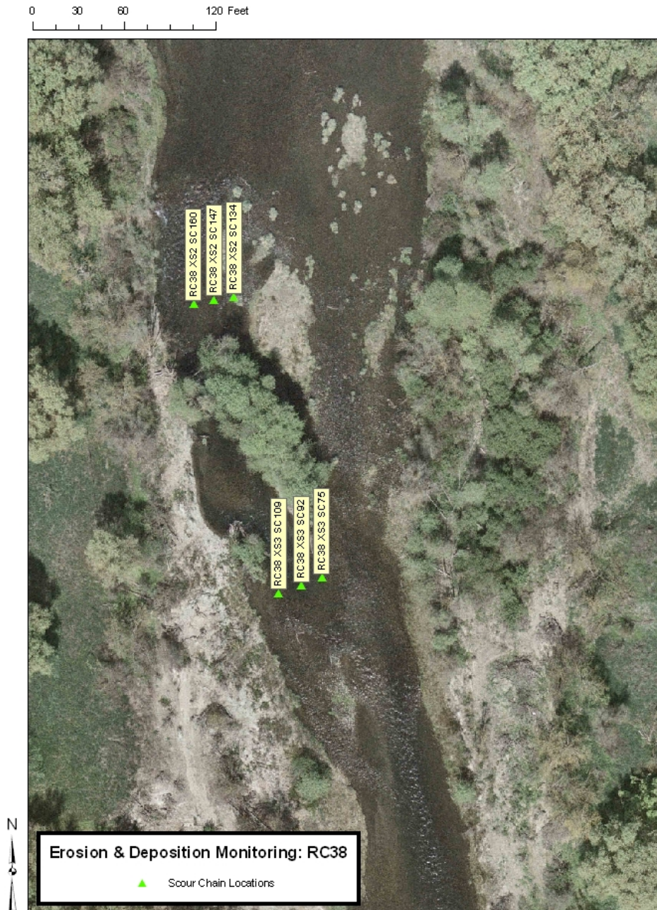
1 2 Figure 7-1: Scour chains locations at RC38. The first installation of scour chains were 3 placed along XS2 and XS3 due to previously observed erosion and deposition in these 4 areas.
