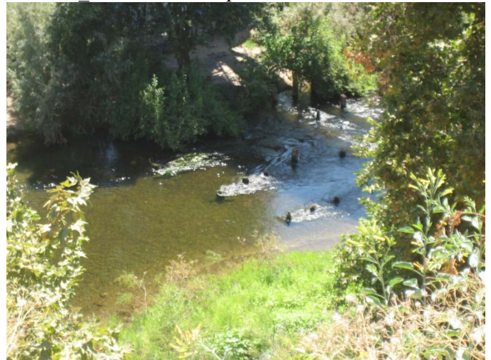
Photo 14_B. Old wooden piers in channel
