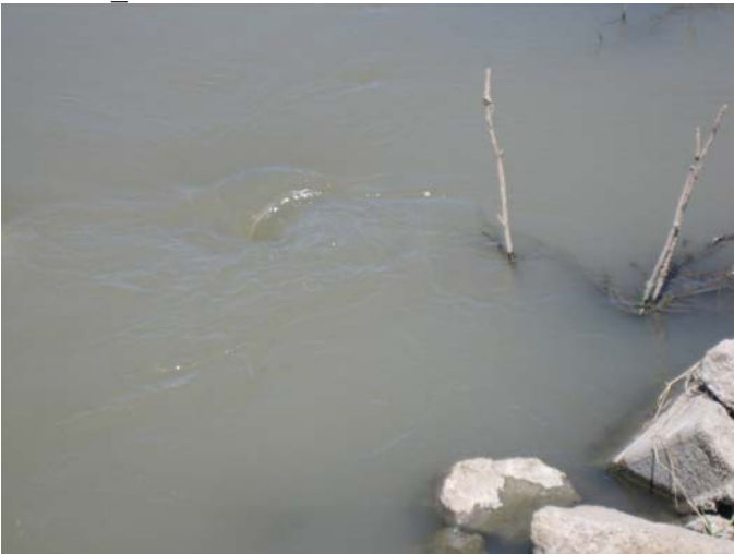
Photo 51_E. Culvert inlet
