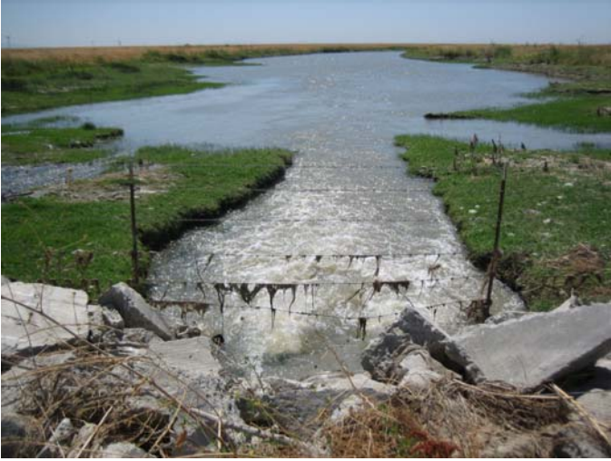
Photo 51_C. Looking downstream from the crossing at the culvert outlet
