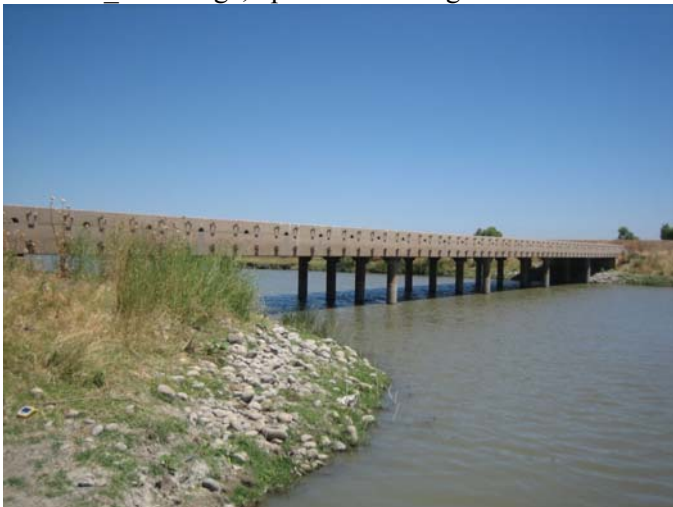
Photo 50_A. Bridge, upstream looking downstream
