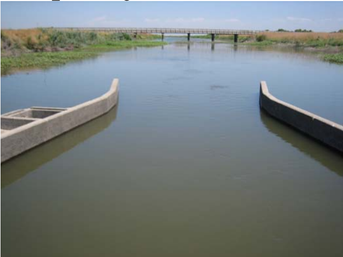
Photo 29_E. Looking downstream from flume
