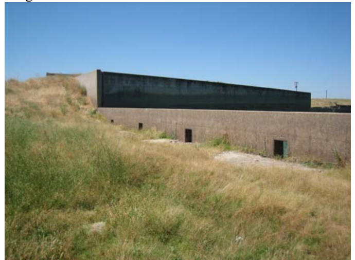
Photo 35_B. Low flow openings looking at left bank and wingwall
