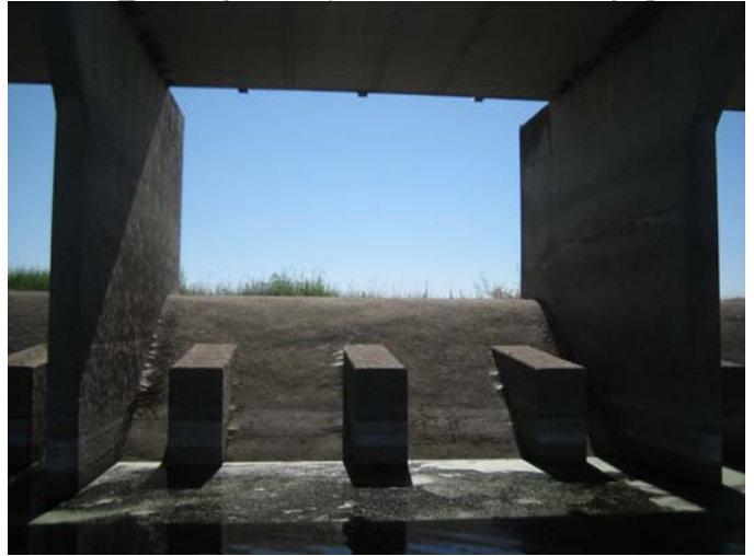
Photo 49_B. Ungated bay, downstream looking upstream
