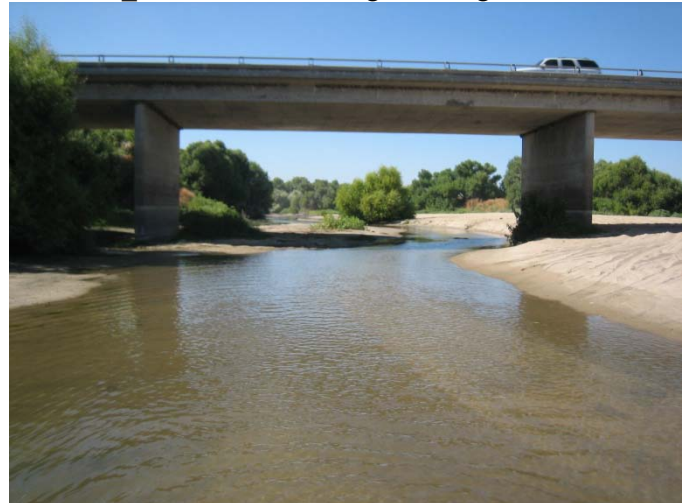
Photos 27_B. Westbound bridge looking downstream
