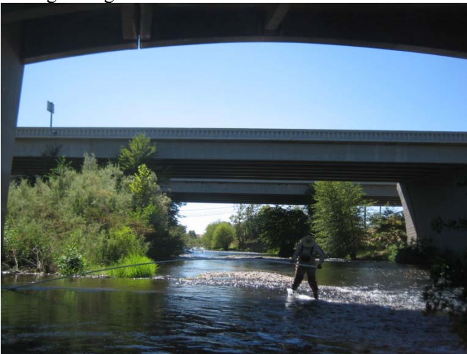
Photo 11_A. Bridges looking downstream from the frontage bridge
