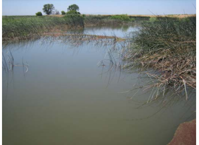
Photo 29_D. Looking upstream from structure headwall
