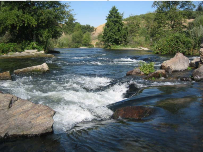
Photo 5 A. Rock weir looking downstream
