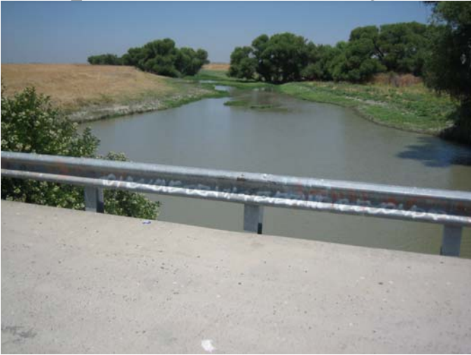
Photo 47_C. Channel downstream from bridge deck
