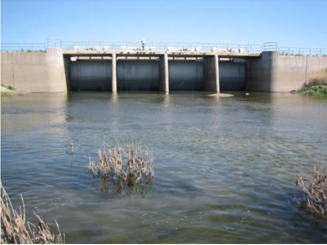
Photo 21_C. Diffusers and gate
