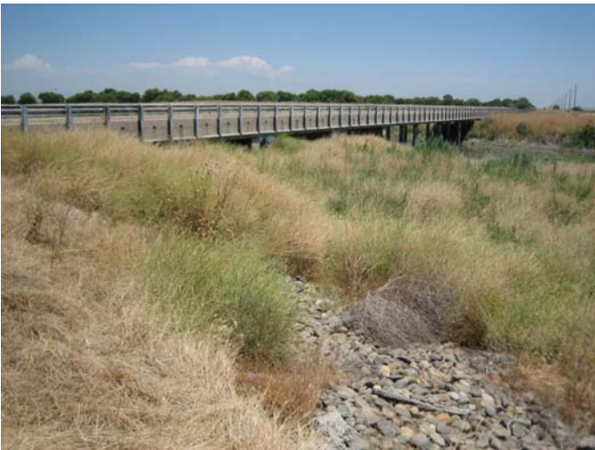
Photo 55_A. Washington Bridge looking downstream
