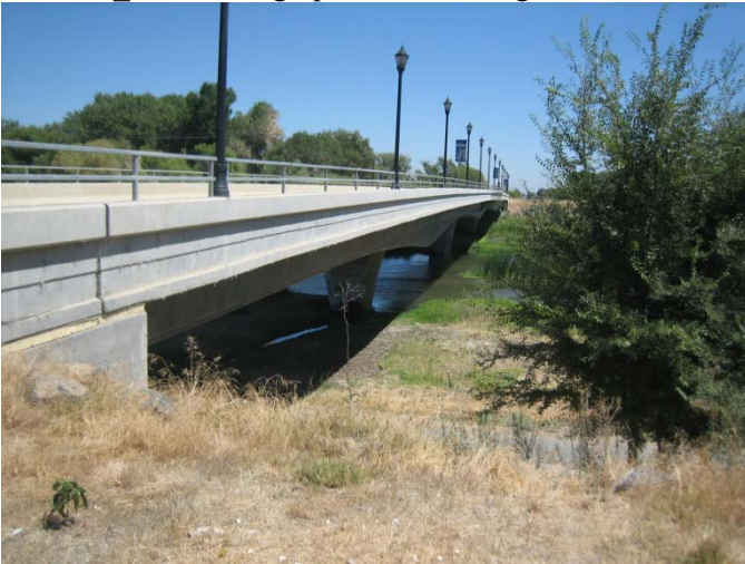
Photo 25_A. Looking upstream at Bridge from left bank
