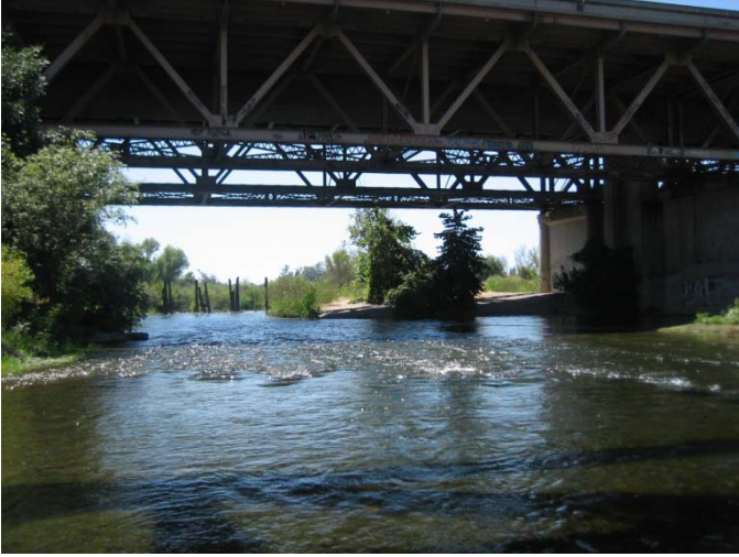
Photo 16_C. Channel upstream bridges looking downstream
