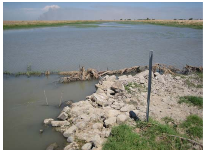
Photo 51_B. Looking upstream from the crossing near the culvert inlet
