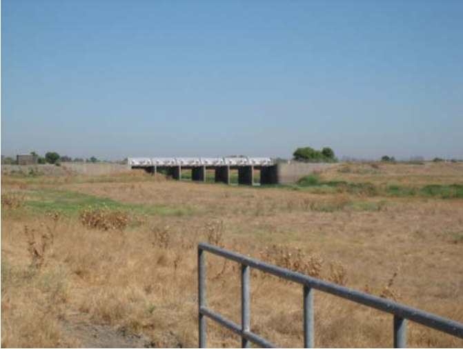
Photo 48_A. Structure, upstream looking downstream
