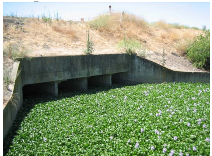
Photo 28_B. Culvert outlets downstream
