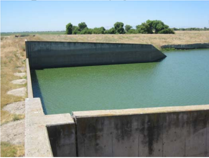
Photo 35_C. Structure looking at pool downstream
