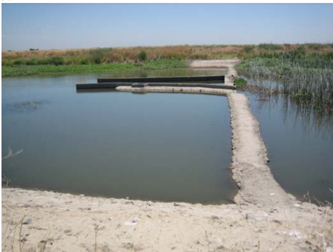
Photo 29_A. Sand Slough Control Structure from the left bank
