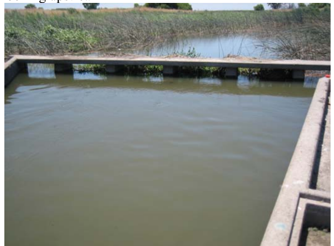
Photo 29_B. Sand Slough Control Structure openings looking upstream
