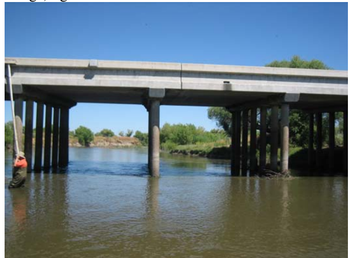
Photos 43_B. Looking downstream at Highway 140 Bridge, right bank
