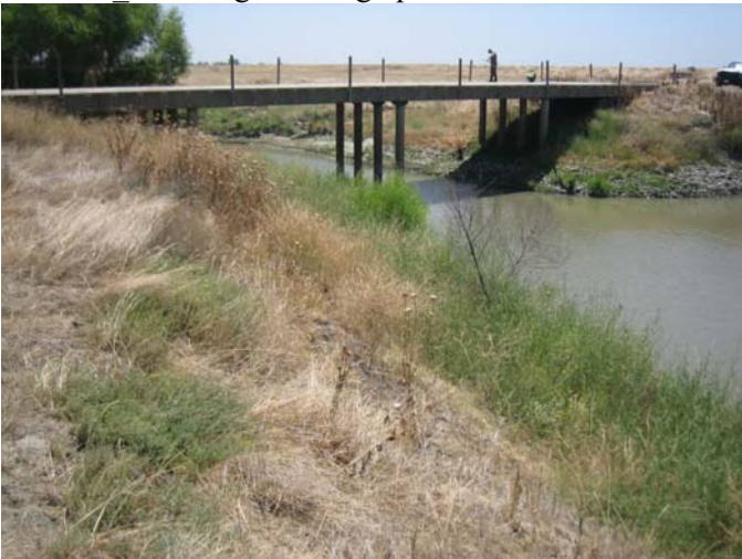
Photo 45_A. Bridge looking upstream
