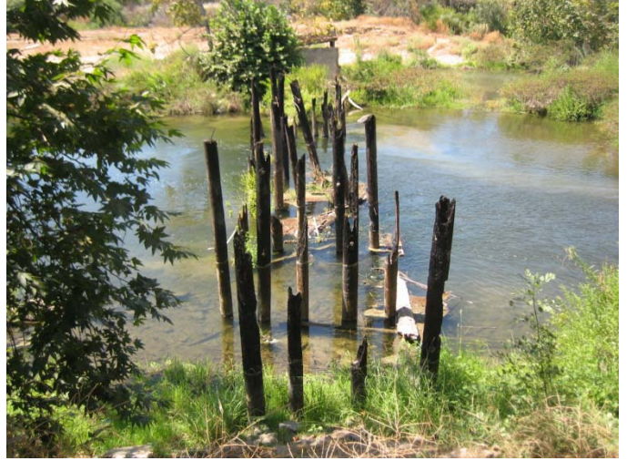
Photo 16_D. Wooden piers from old crossing
