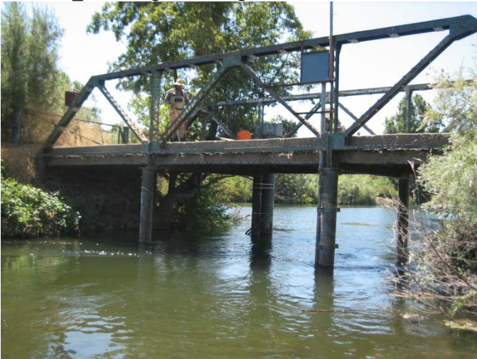
Photo 17_A. Bridges looking downstream
