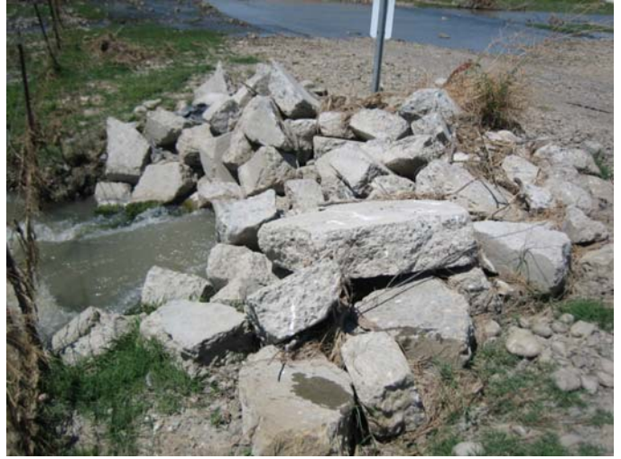
Photo 51_D. Culvert outlet
