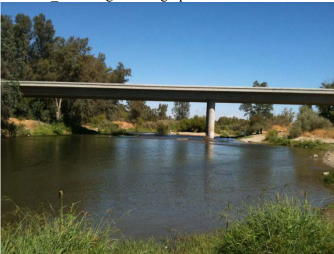
Photo 18_A. Bridge looking upstream
