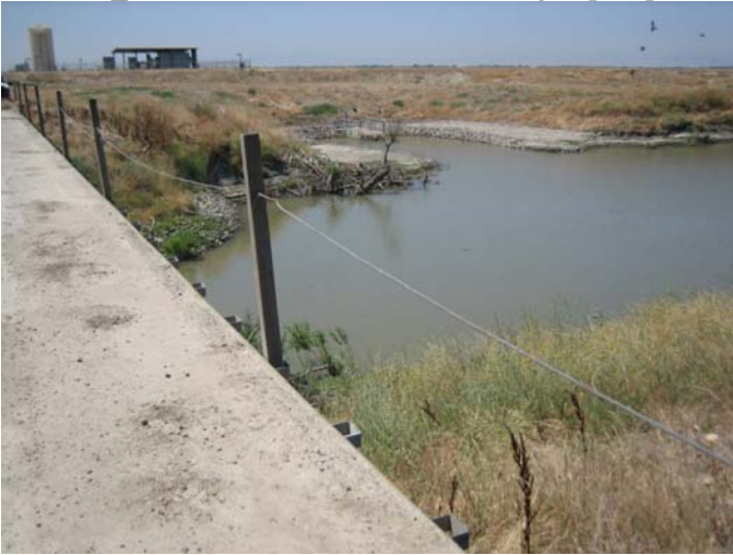
Photo 45_C. Channel downstream looking at pump
