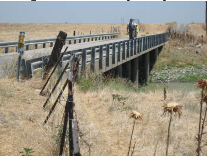
Photo 47_A. Greenhorn Road bridge from right bank
