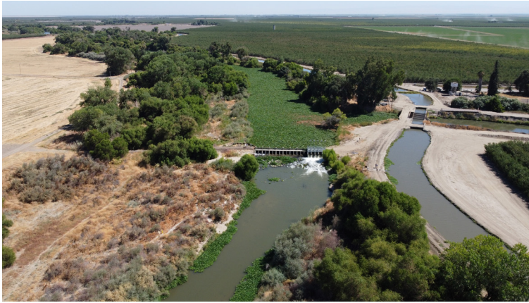
Existing view of Sack Dam and Arroyo Canal facing south.
