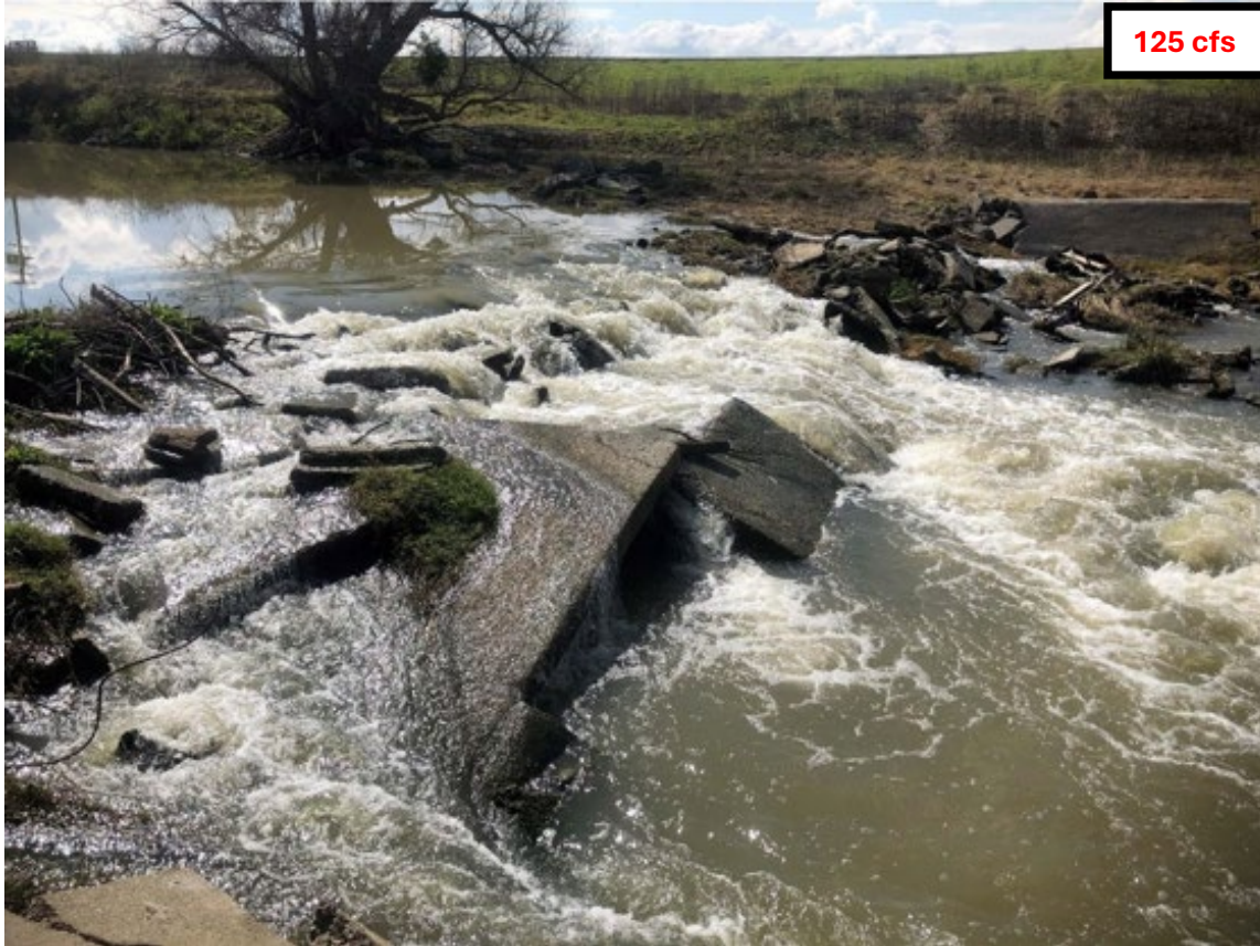
Figure 6. Photograph Date 3.19.2020 11:31. QA/QC: EBM: 77 cfs daily avg, SJS: 239 cfs daily average. C. Moore estimate approx. 125 cfs instantaneous.
