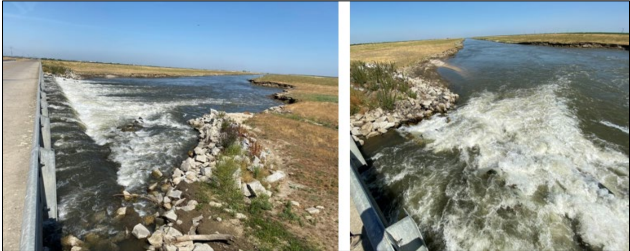
Figure 4 Avenue 21 Bridge. (Left) Photo taken from the right showing a potential fish passage route along the right bank where the drop appeared lower. (Right) Potential fish passage route along the left bank where the drop also appeared to be lower.
